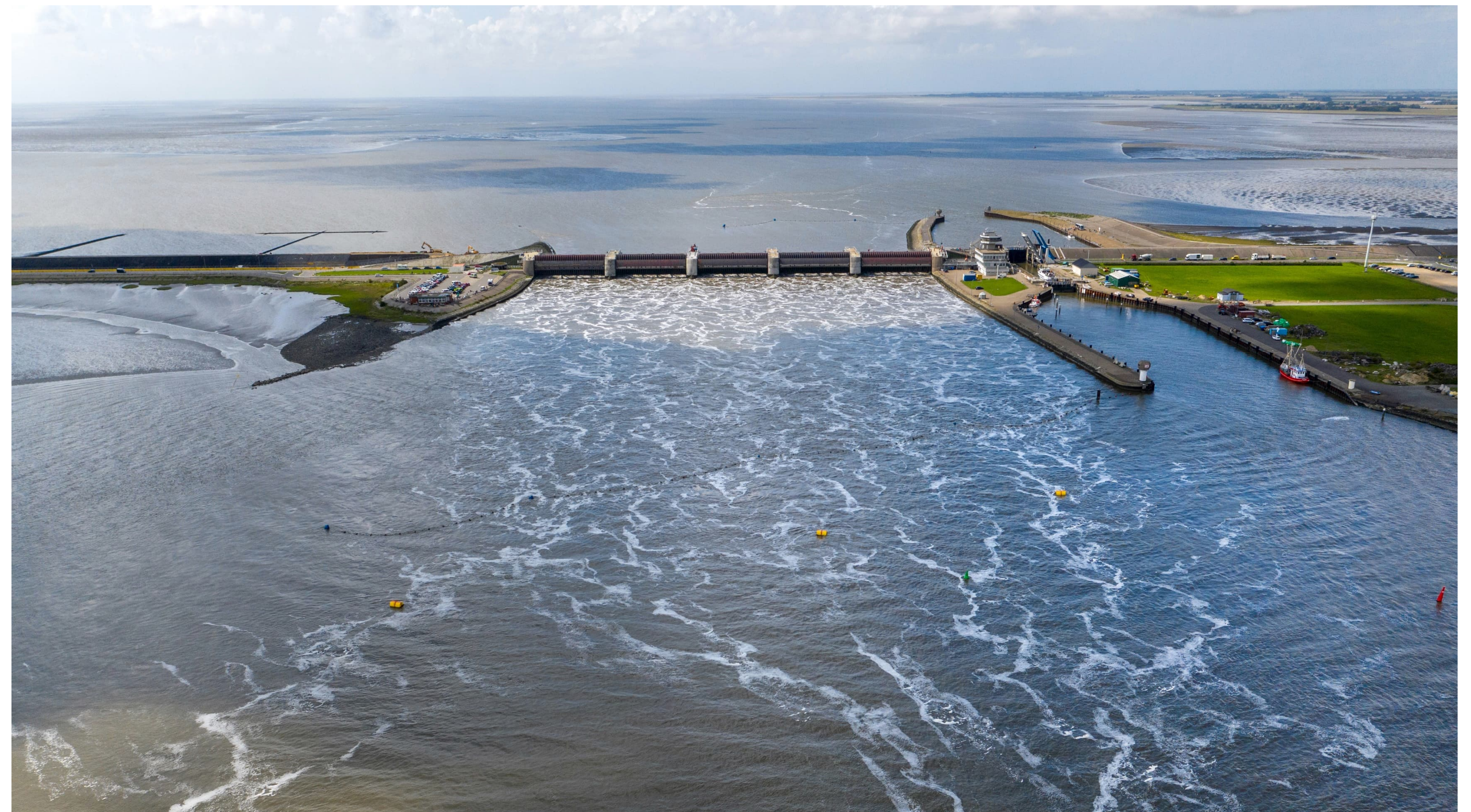
Fig. 4: Aerial photograph of the storm surge barrier of the Eider
